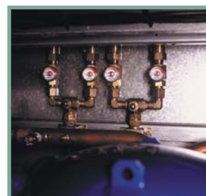
Dual pressure relief valve
